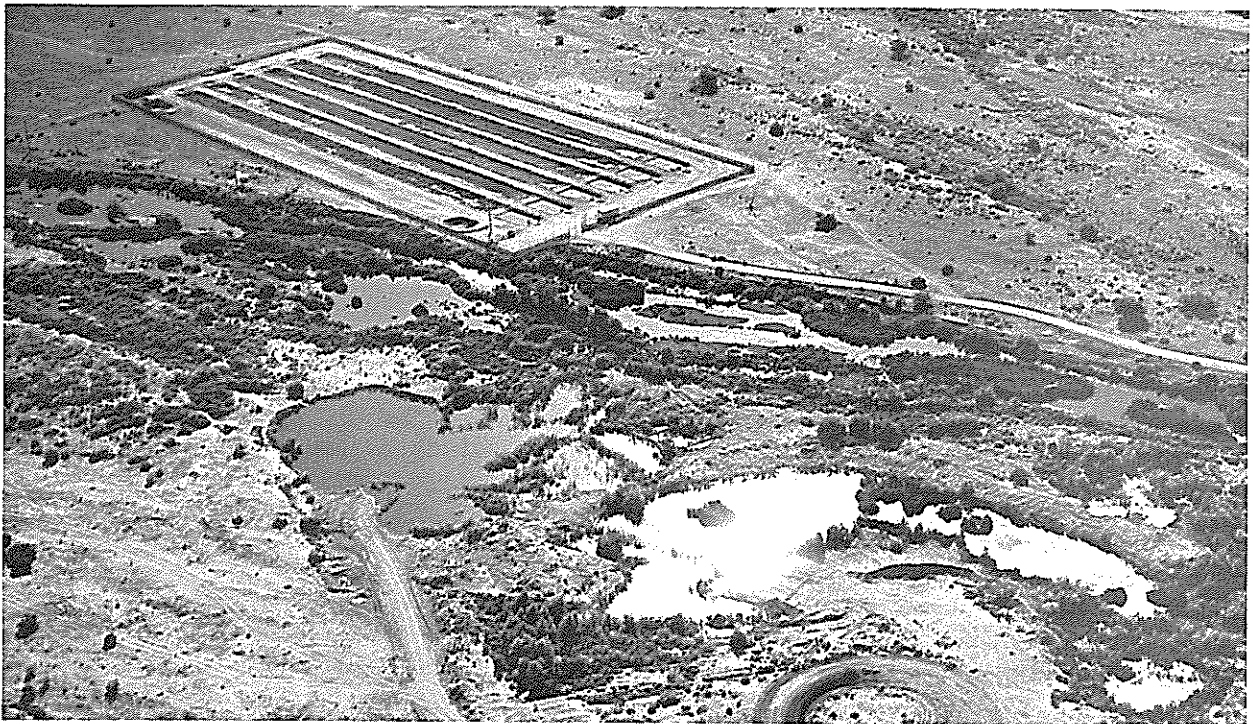
Infiltration basins with bermuda-grass and flume for recording outflow (foreground).
